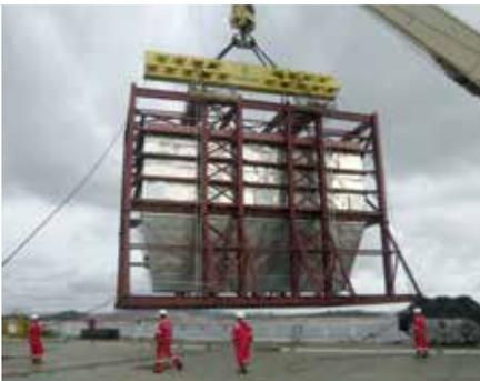
Loading coal mill baghouse with 180 tons and 14-meter height at Batam Anchorage ex barge to MV Jumbo Javelin
