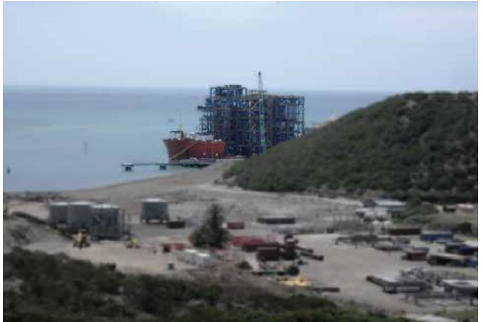
Dockwise's MV Trustee berthing at Vavouto carrying four of the 18 large onshore modules ex Qingdao to New Caledonia
